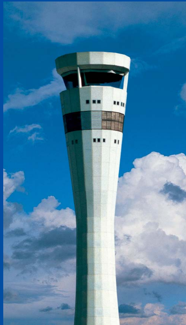
The Control Tower
