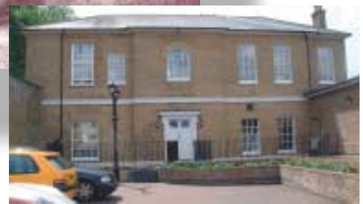
New - Today the station building is home to a high tech marketing company.
